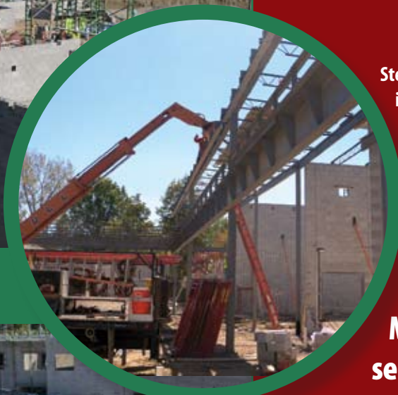
With Stafford Elementary in the background, workers install the decking before beginning work on the second floor of Milkovich.
