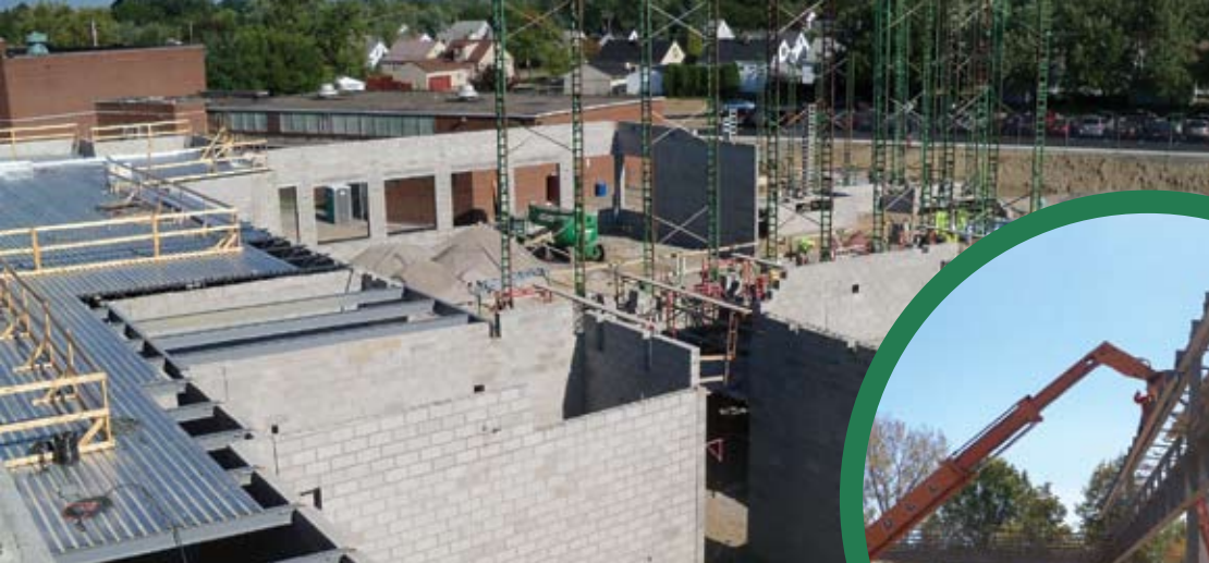
With Stafford Elementary in the background, workers install the decking before beginning work on the second floor of Milkovich.
